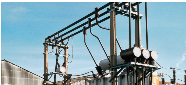
GASLINK® SF 6 insulated busbar system
